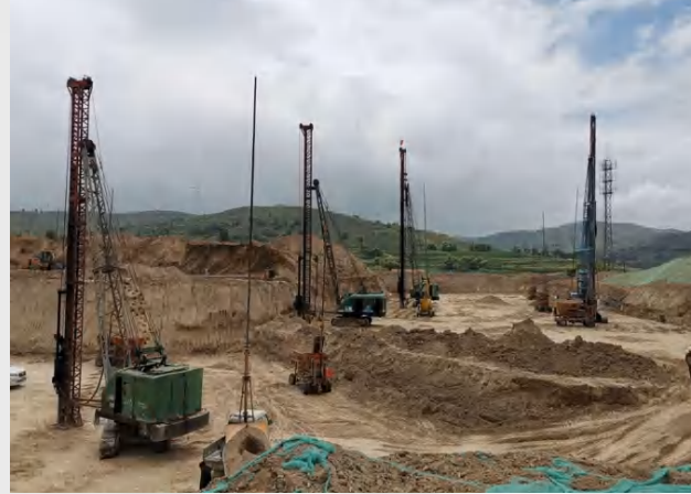
Field Construction Site
